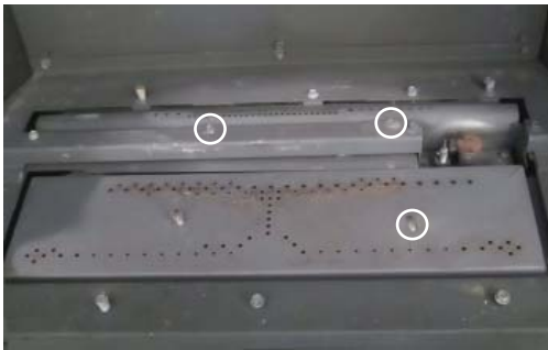
1. Remove the three screws from the rear log support and burner as shown.
